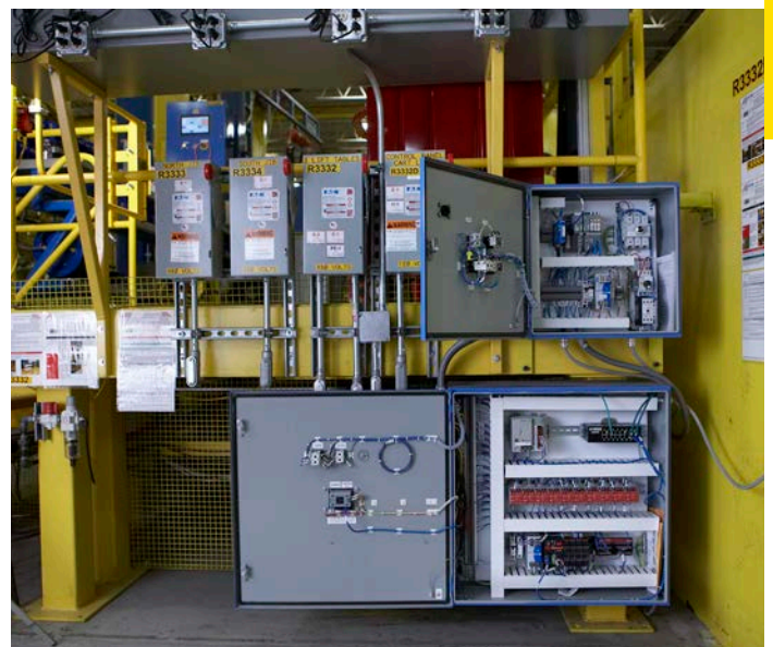
Figure 7.6.5.a Existing installation labeling per 240.86(A) and 110.22(B).
